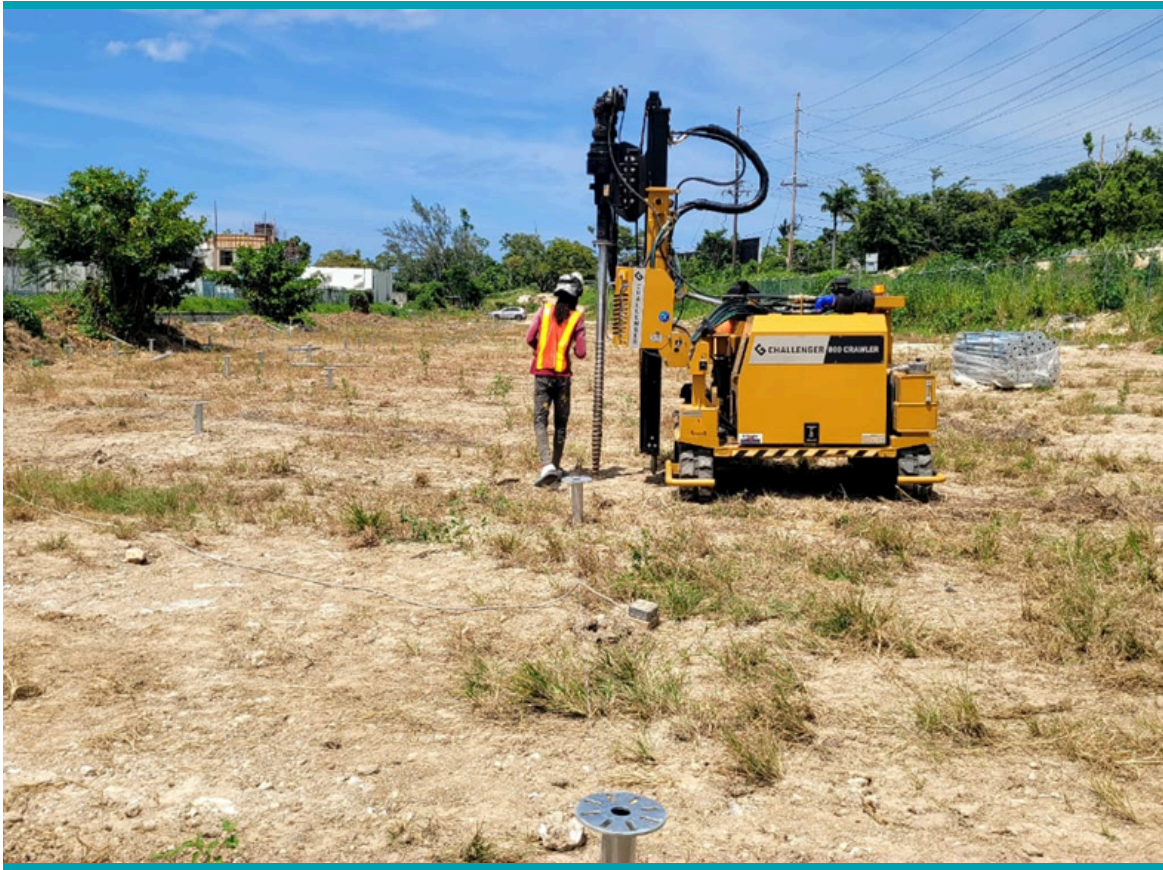
Screw Pile Installation - Phase 3 Solar System Ground Mount
