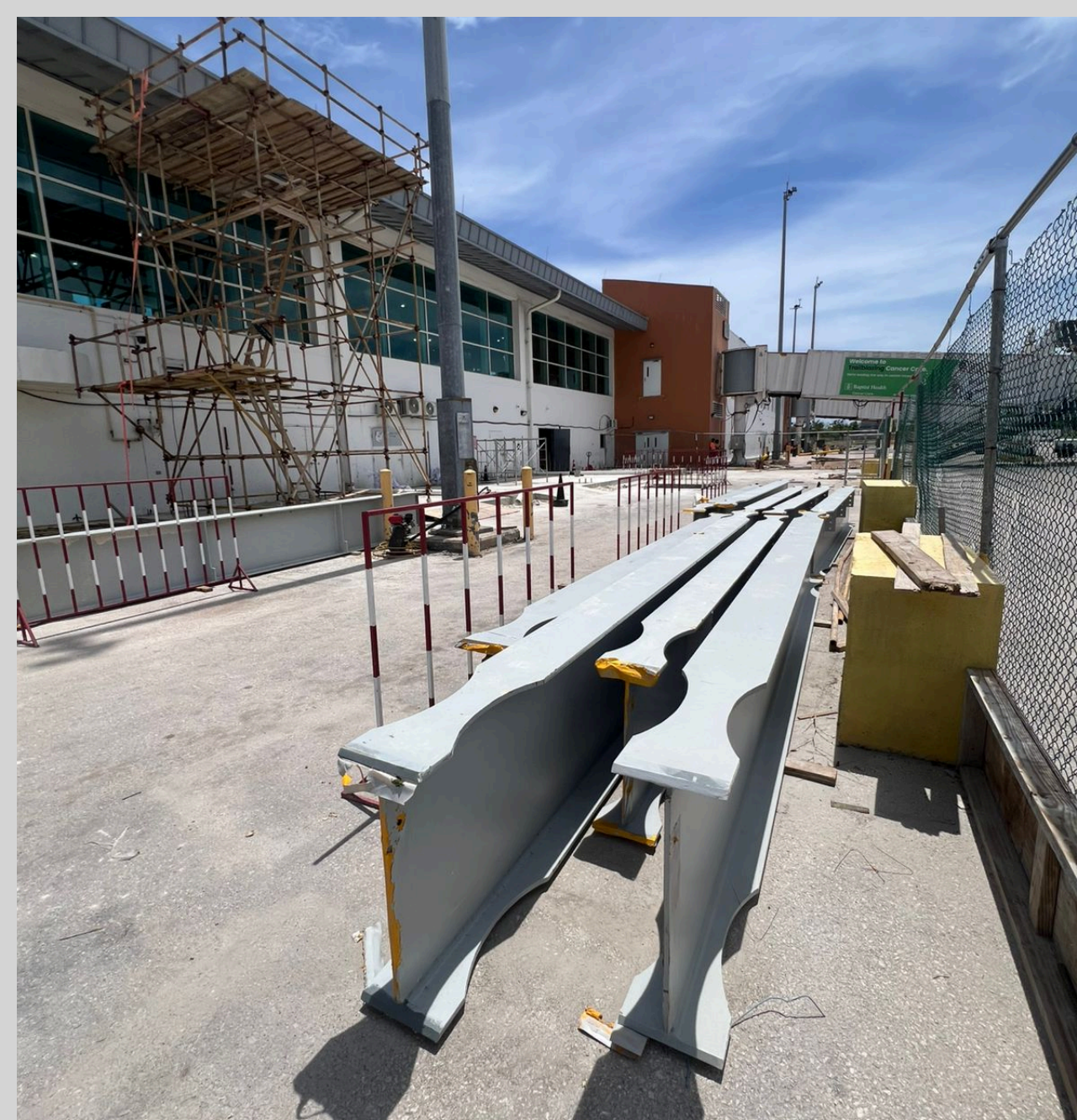
Steel delivered to site
