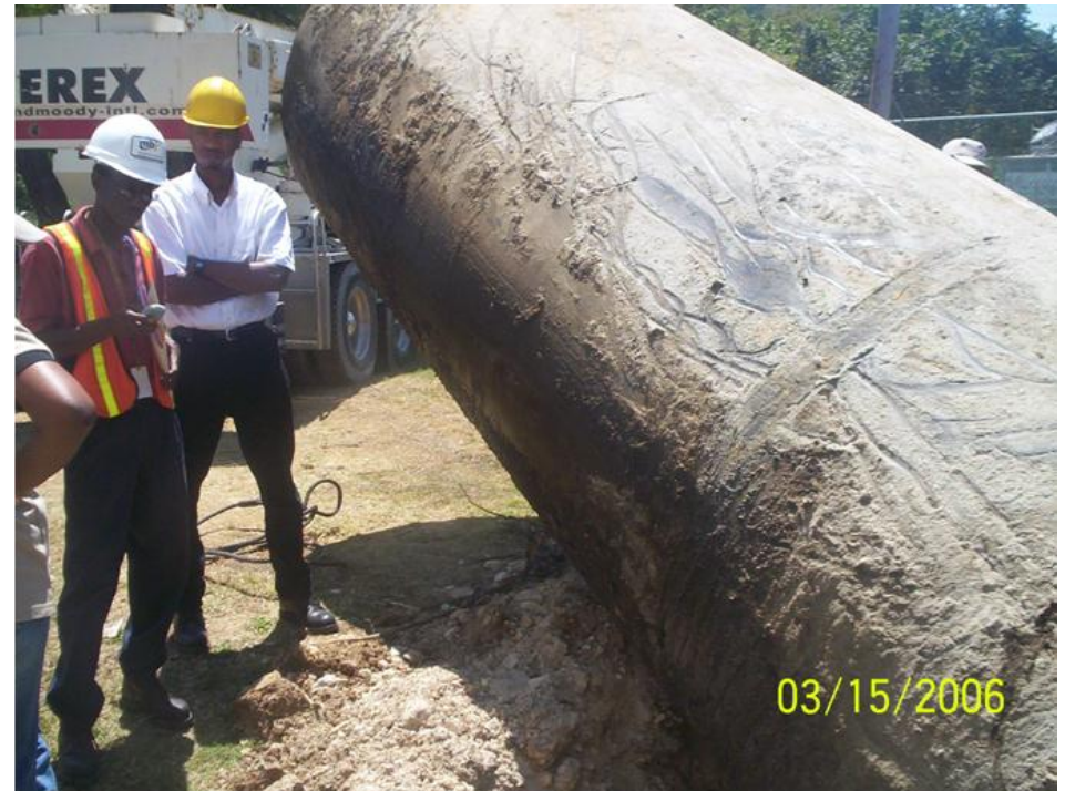
Decommissioning of diesel underground storage tank (UGST) at MBJ Electrical Main Substation
