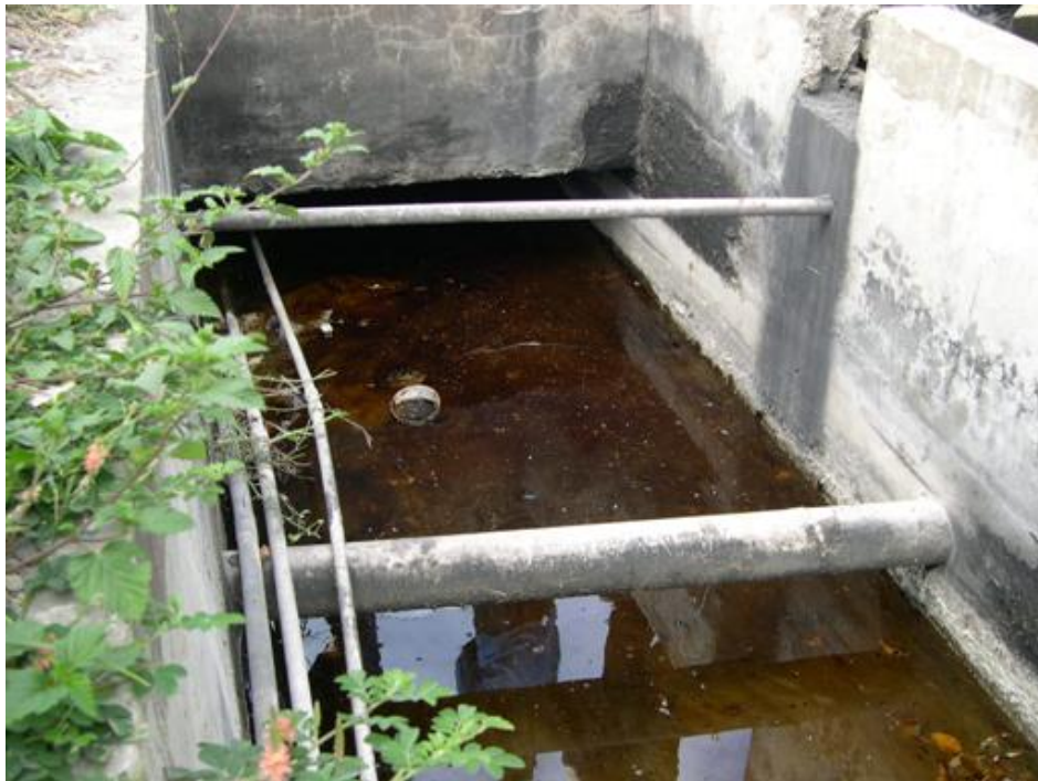
Contamination of storm drain due to leakage from a diesel underground storage tank (UGST) at Texaco Service Station
