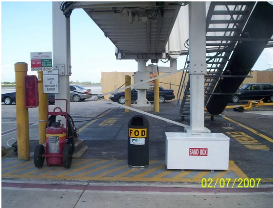
Spill/Fire response supplies are at each passenger boarding bridge on the ramp
