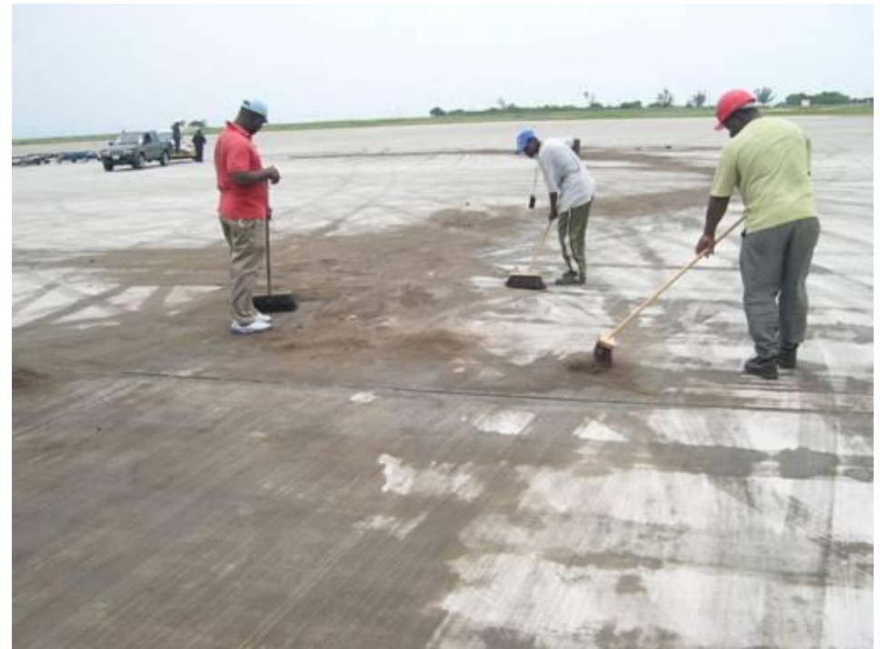
Fuel spill clean-up carried out by MBJ Maintenance & Engineering Department
