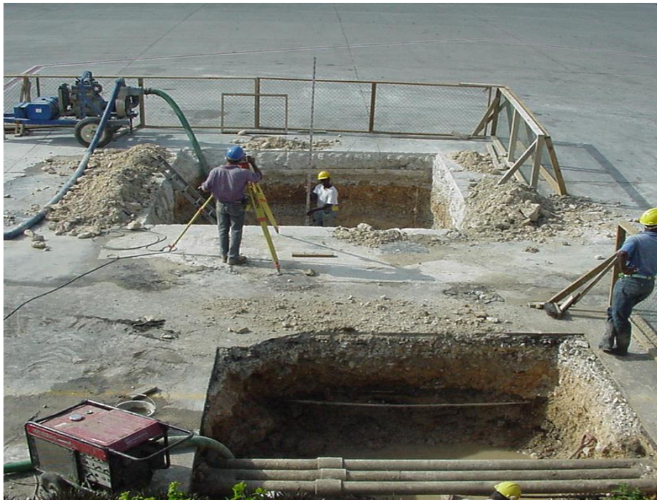
Contamination from former fuel hydrant system discovered during excavation for the footings of a passenger boarding bridge
